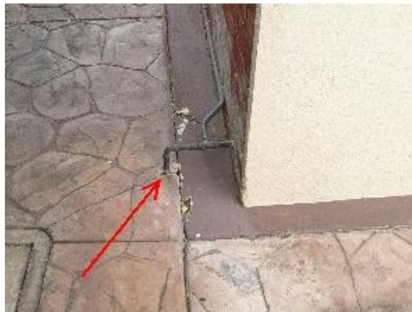
Perimeter paths Trip hazard Safety Hazard Type: F Water piping by rear corner of toilet is a trip hazard.
